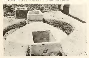
Installation for converting wastes into methane.
